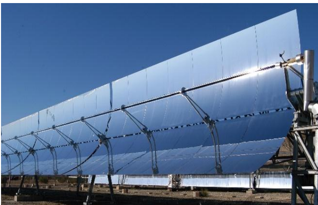
Figure-6. Parabolic-trough solar collector at Plataforma Solar de Almería in Spain [20].
