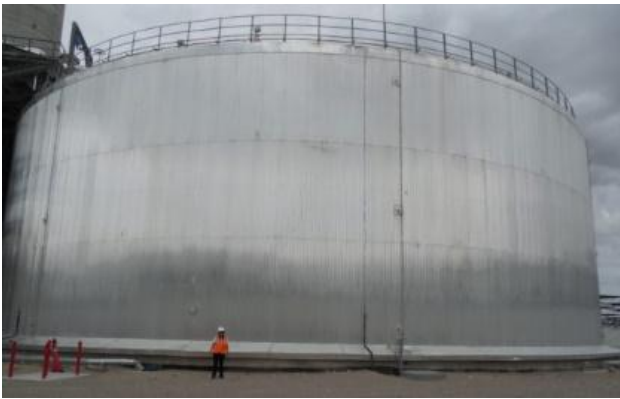
Figure-4. The (TES) tank at the Crescent Dunes in Nevada holds molten salt at 565°C [10].
