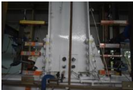
Figure 13. Documentation LVDT Transducer Installation.
