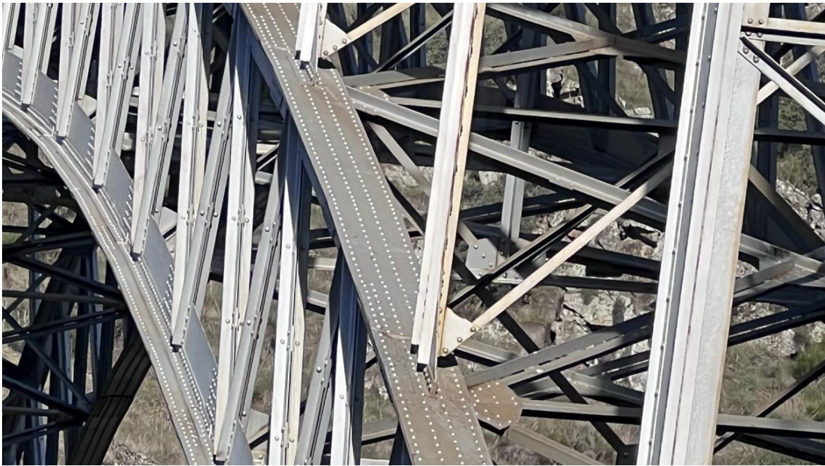
Figure 10. Examples of upright supports on the arch, using gusset plates fastened with bolts, on the upstream side.
