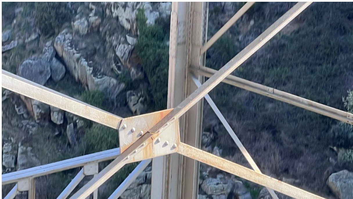
Figure 17. Localized corrosion on one of the braces of the sheet pile walls at the western end of the bridge, upstream side.
