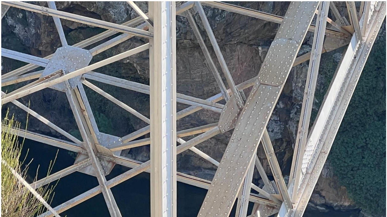
Figure 19. General state of the arch, in a section between support uprights.
