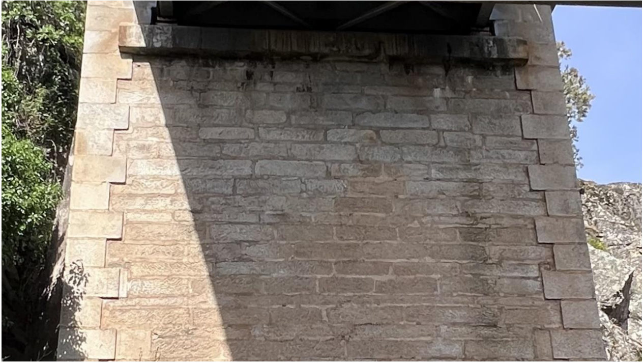
Figure 13. Wall of the second abutment with runoff water traces.
