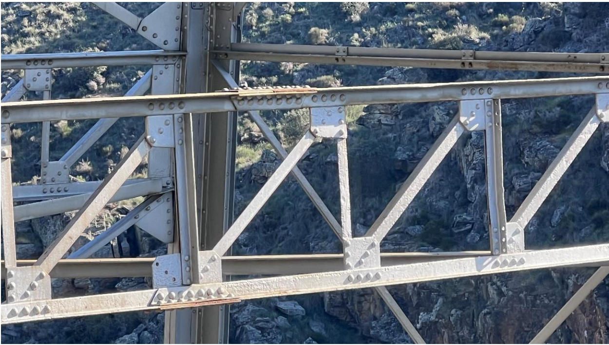
Figure 20. Detailed view of an arch section with localized corrosion at connection points.
