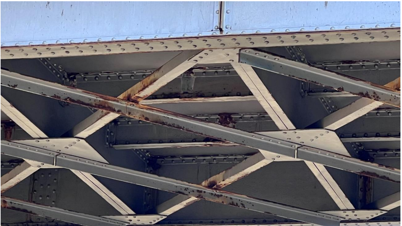
Figure 23. Detailed view of a deck section with localized corrosion on several elements.
