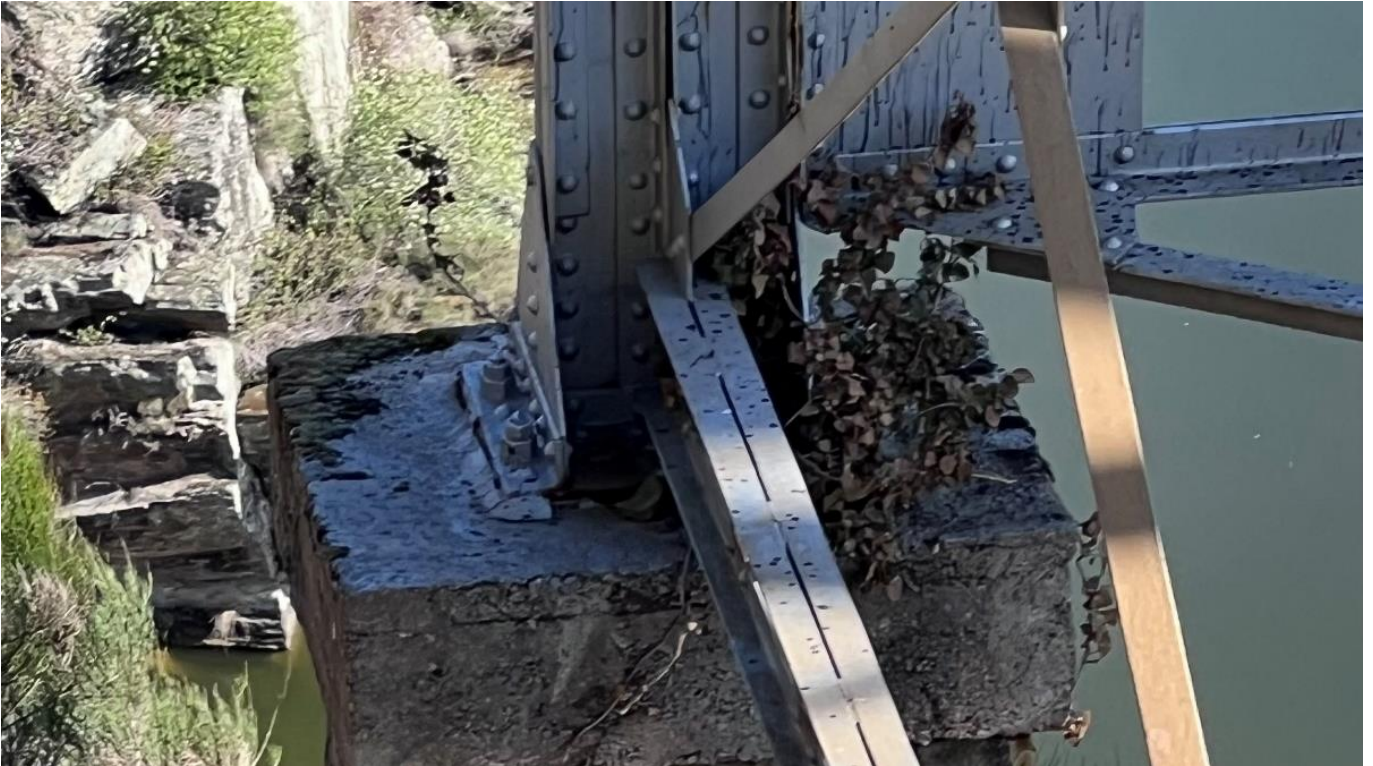
Figure 14. Presence of organic matter and vegetation on the concrete footing of sheet pile wall 6, downstream side.
