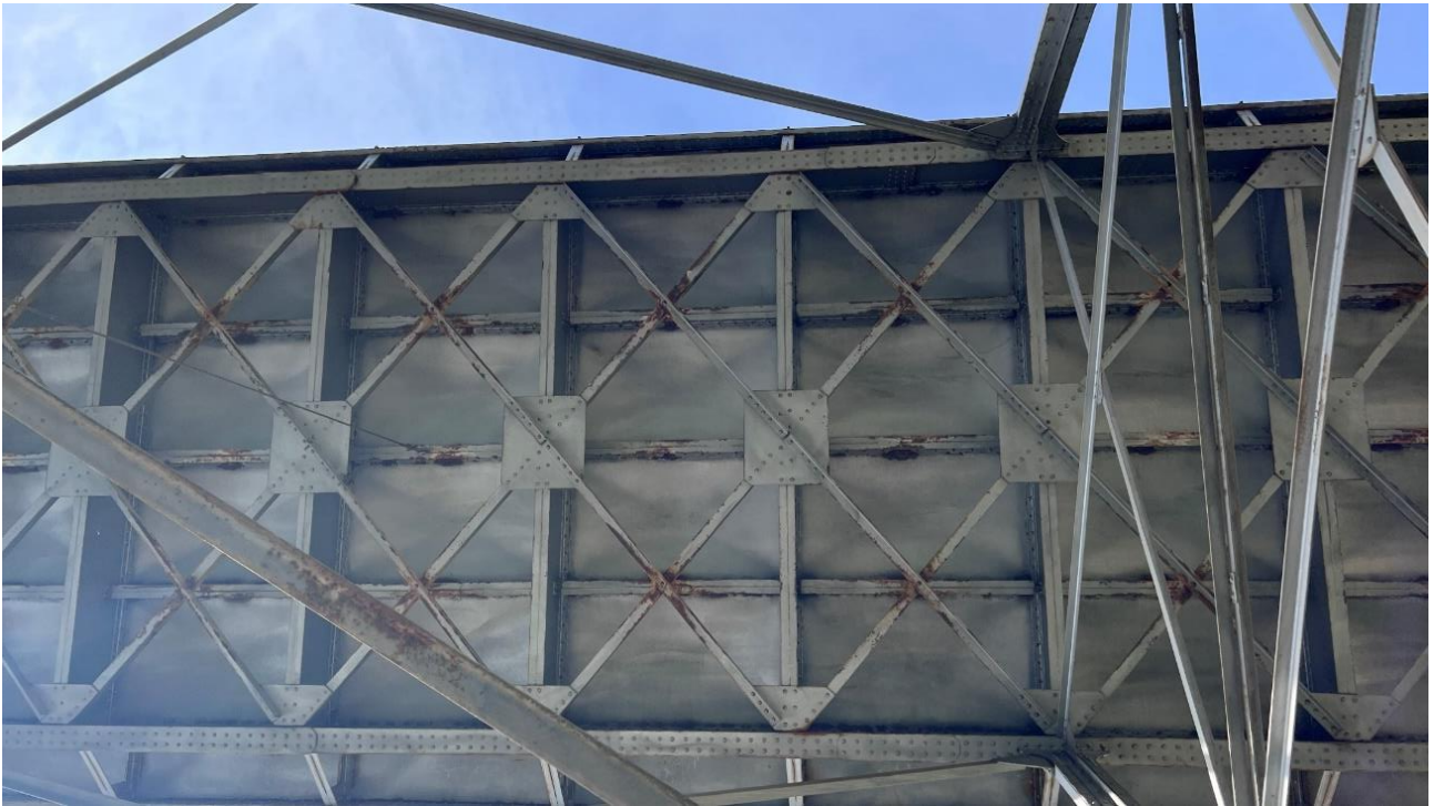
Figure 22. Bottom view of a deck section, showing numerous elements with localized corrosion symptoms (photograph by the author, taken with a drone).
