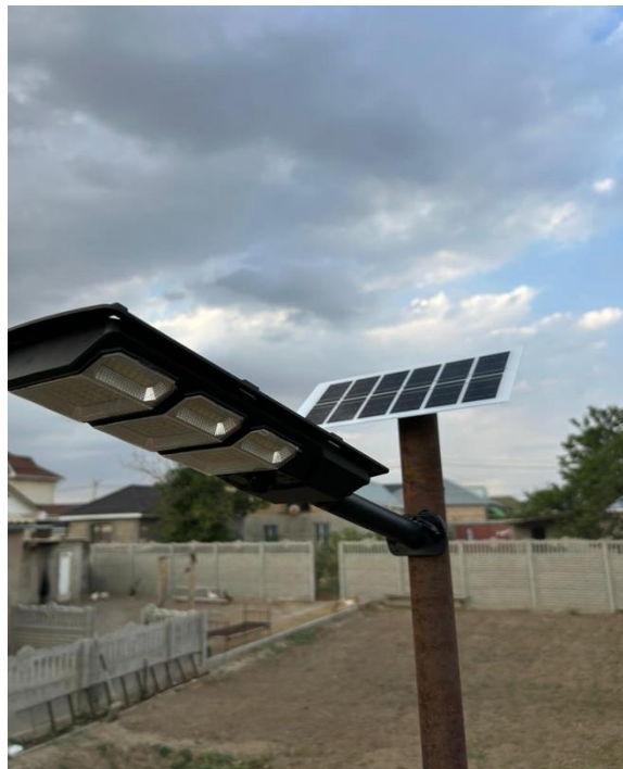
Figure 4. Solar street lamp with a housing made of AD31 aluminum alloy.
