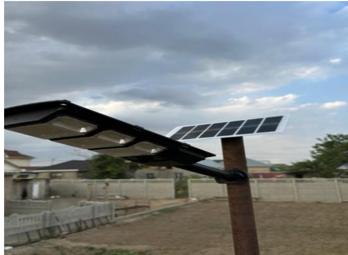
Figure 2. Lantern with solar panel made of aluminum alloy AD31.
